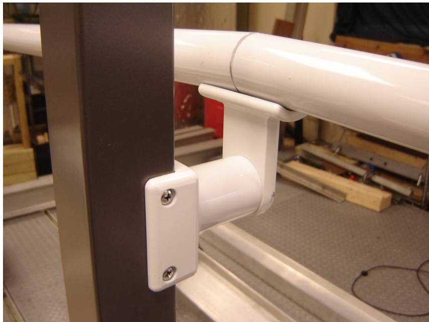
Photo No. 6 Mid-Rail Bracket, Spacer Tube, and Small Post Adaptor
